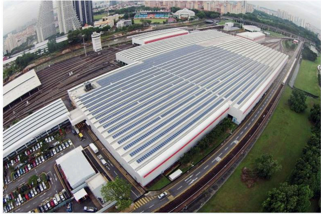
Microsoft yesterday said it will buy 100 per cent of the electricity generated from Sunseap's 60 megawatt-peak solar power project for 20 years for its Singapore data operations. Sunseap has solar panels on hundreds of rooftops across Singapore. PHOTO: SUNSEAP
